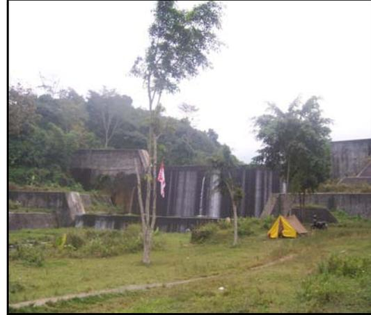
**Gambar 10** Bendung Penahan Sedimen K. Jari
