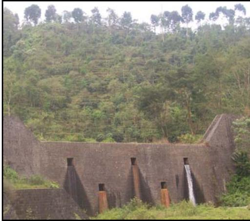
**Gambar 9** Bendung Penahan Sedimen K. Jari
